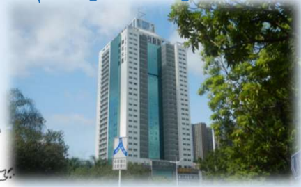
ALLY Engineering (ShenZhen)
